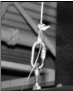
Figure 8: Wire rope detailing suspension or seismic tether
